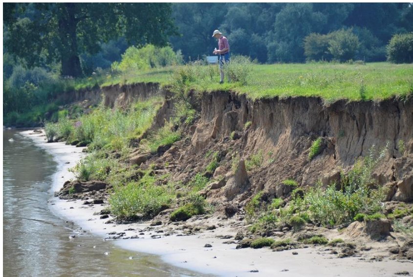
Figure 3.28: The regulated Meuse River near Gennep, the Netherlands, where cohesive banks present a shallow submerged terrace and vegetation naturally growing after a few years
