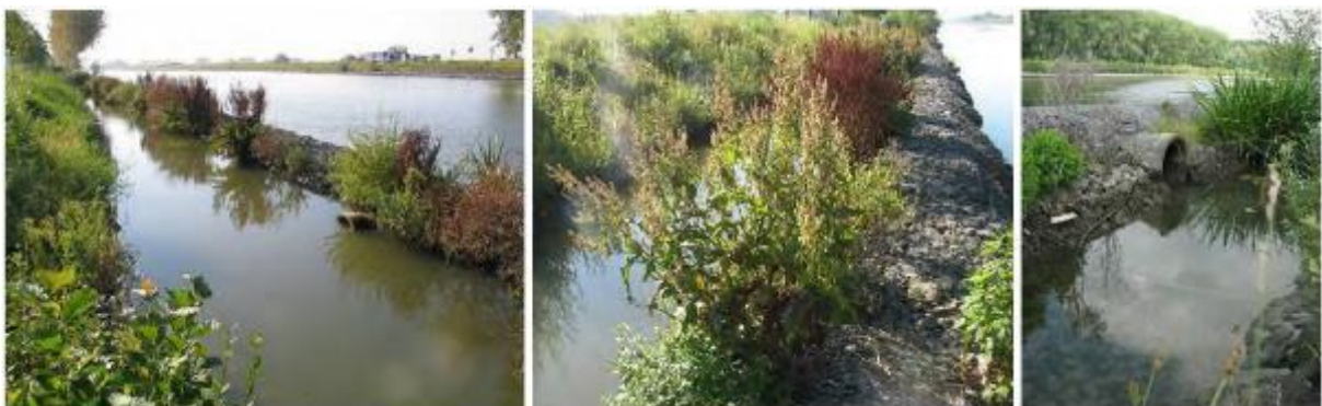
Figure 3.4: Canal Brussels-Scheldt, Belgium Quarry stone parallel dam with underwater openings
