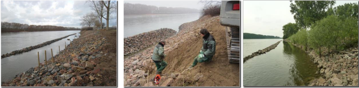
Figure 3.14: Vegetated rip rap after installing cuttings and log-branch cuttings (left), while installing hedge layers (middle), some months after installation (right; Rhine km 440.7)
