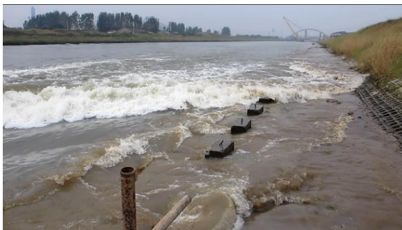
500 t ship in the test section (high water level)
