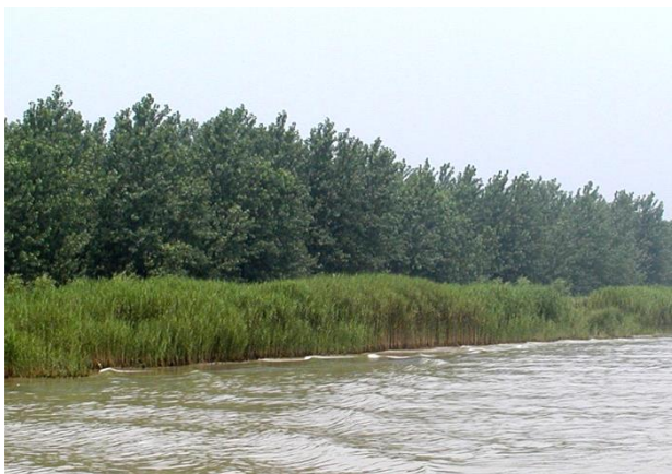
Figure 3.12: Bank protection with reeds along the Huai'an-Huaiyin section of Beijing-Hangzhou Canal, China
