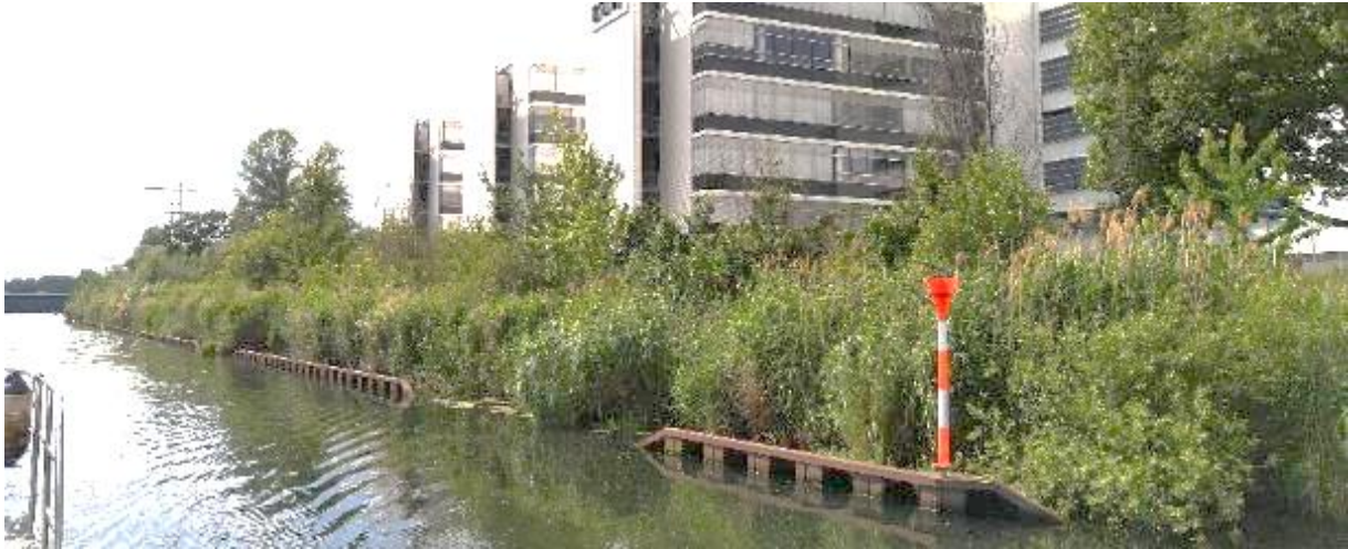
Figure 3.2: River Spree at Berlin-Charlottenburg, Germany Top level about 0.3 m above MW; Sill level at openings about 0.8 m below MW
