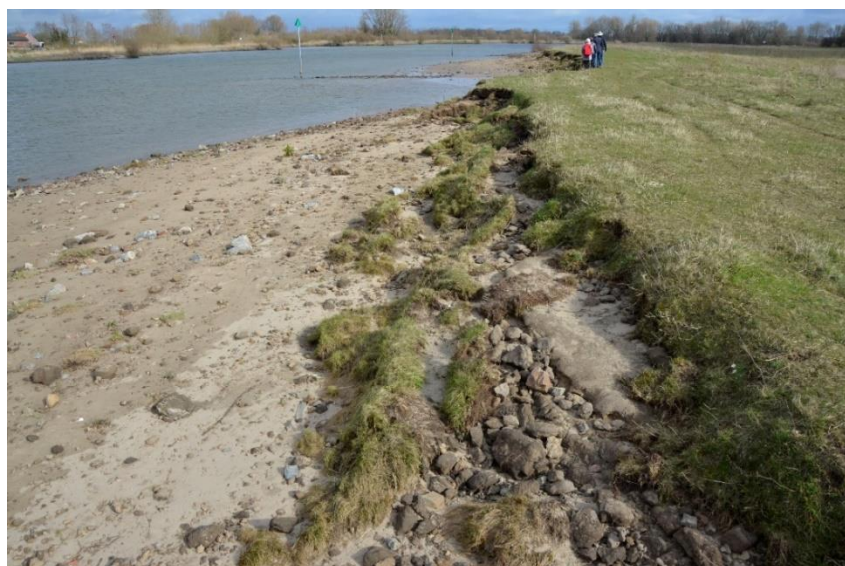
Figure 3.29: Brussels-Scheldt Canal, Belgium, quarry-stone parallel dam with underwater openings
