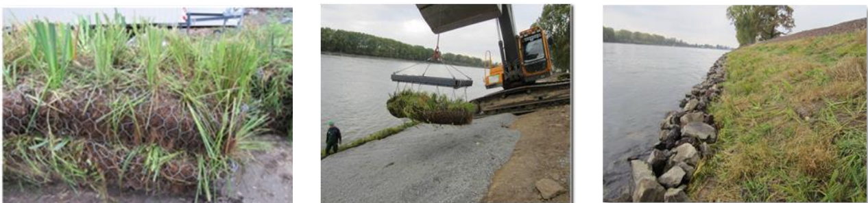
Figure 3.15: Reed gabions (before, during, and after installation)
