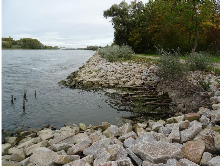
Figure 3.27: Fish shelter made of deadwood on the River Rhine near Daxlanden in October 2019 (Photo: S. Wieland, BfG)
