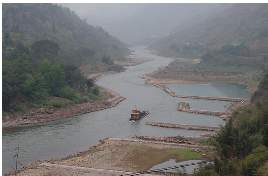
Figure 3.37: L-head groyne works in the Chishui River, a tributary of the upper reaches of the Yangtze River (with ecological benefits)
