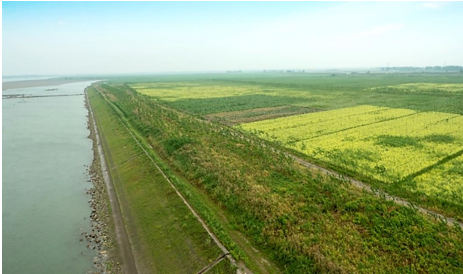
Figure 3.36: Ecological protection of banks in the middle reaches of the Yangtze River, China
