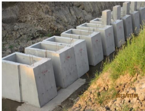
(c) Picture of construction site
