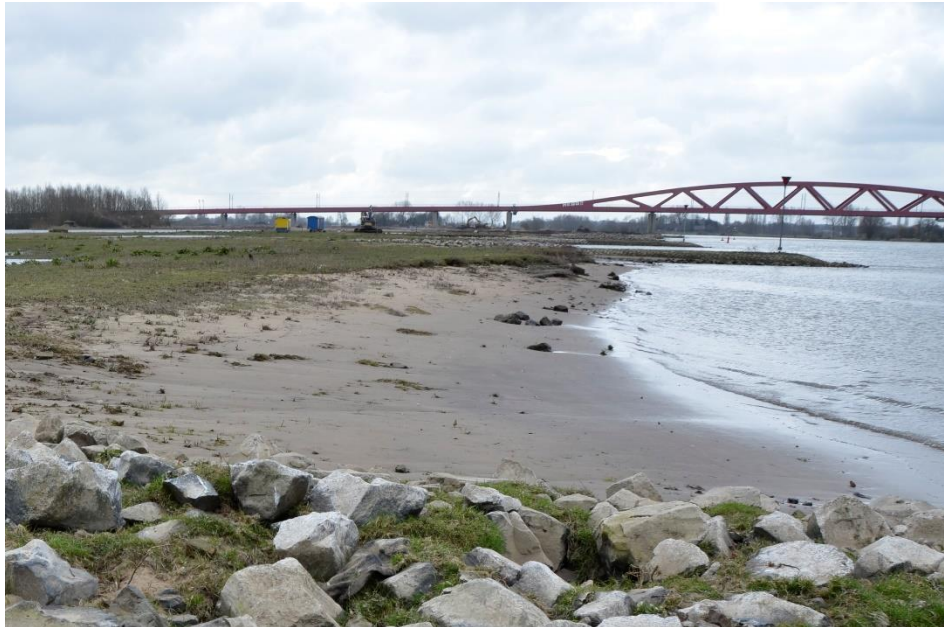
Figure 3.30: The unregulated IJssel River in the Netherlands, with unprotected composite banks between transverse groynes near Zwolle, in the long term
